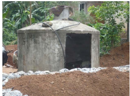
Figure 3.1: Abandoned Rain Water Harvesting Structure, Peruvampadam ST Colony
